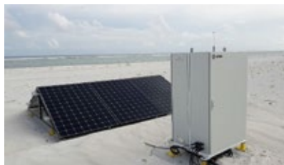
SOLAR POWER SUPPLY
